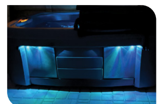
INSIDE & OUTSIDE PERIMETER LIGHTING
